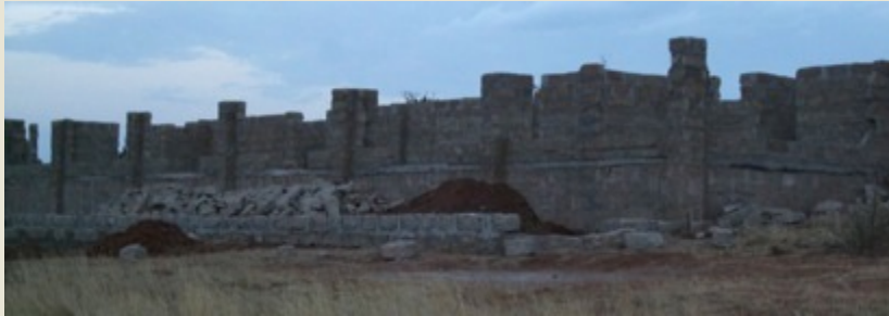
Oct. 2009 – Guest House construction
